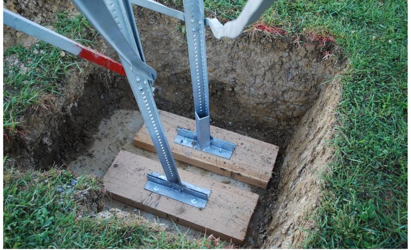
The alignment was accomplished through scooting the legs and anchors using steel pry bars. “Setting the base” was very important before the towers had reached heights of 74 or 87 feet and often more. The Indiana Bilby was set in concrete. In normal tower construction, the anchors were buried in dirt. In some cases, all that secured the anchors to terra firma were sand bags.
