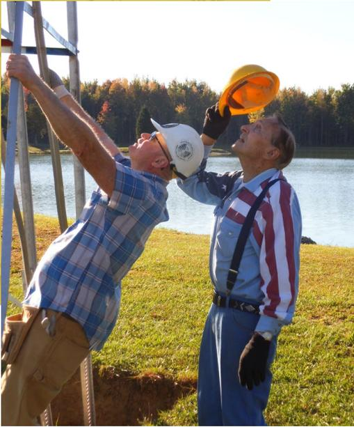
Joe Lindsay and Ulis Jones (retired USC&GS/NGS), both experienced tower builders and observers correct the alignment of the base. By sighting through the intersection of the diagonals (the midpoint of the horizontal ties) up through the tower, the foreman would direct the crew members to adjust the alignments of the inner (red) and outer (blue) towers.
