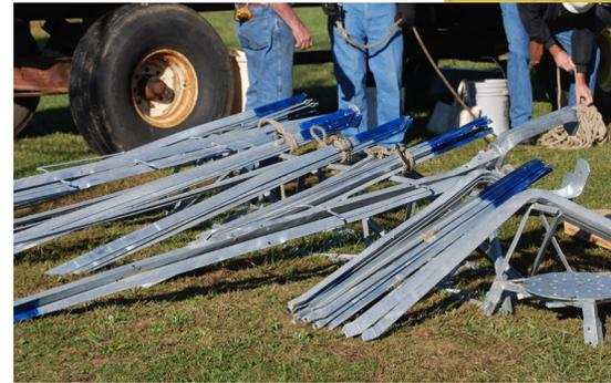
The blue (outer tower) pieces on the ground that will be assembled to become the observation platform and the light tower above. The many, many pieces of the tower were organized and assembled with no directions or guide, but only through the memories of this remarkable gathering of geodetic surveyors.
