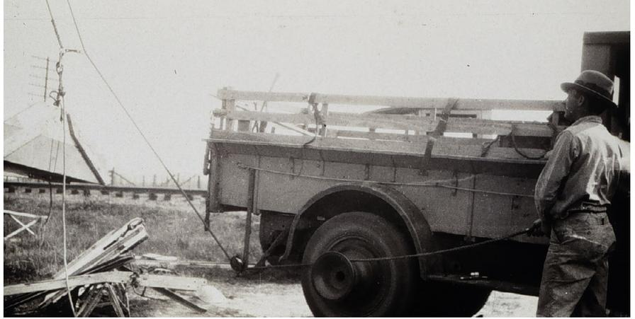
Manpower was specified and economical on the original tower crews. This ingenious method was designed to winch the heavy steel and other parts to the higher sections of the tower. Later designs of this method included a throttle within the rear fender of the haul truck so the rigger could control the speed of the payload on its way up.
